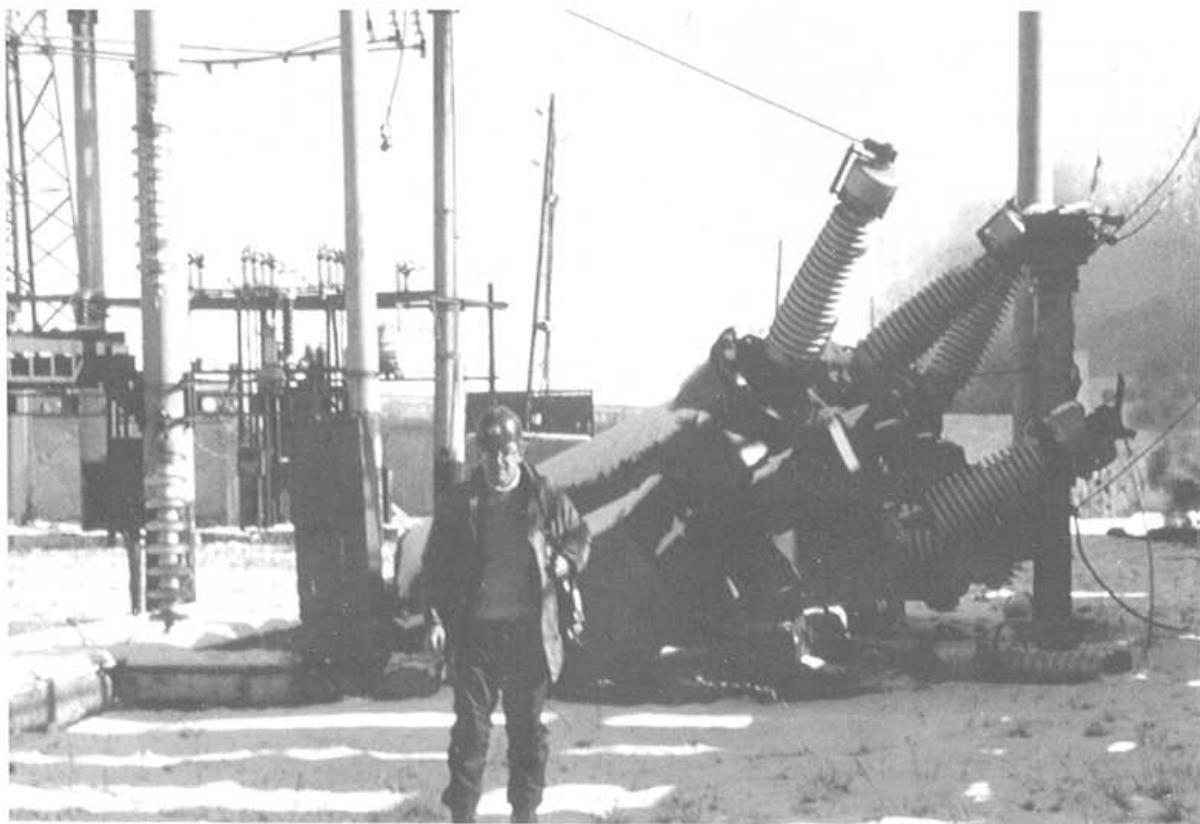
Nalband Electric Substation: The elevated concrete footings of these three oil-filled circuit breakers failed and the units toppled to the right.
