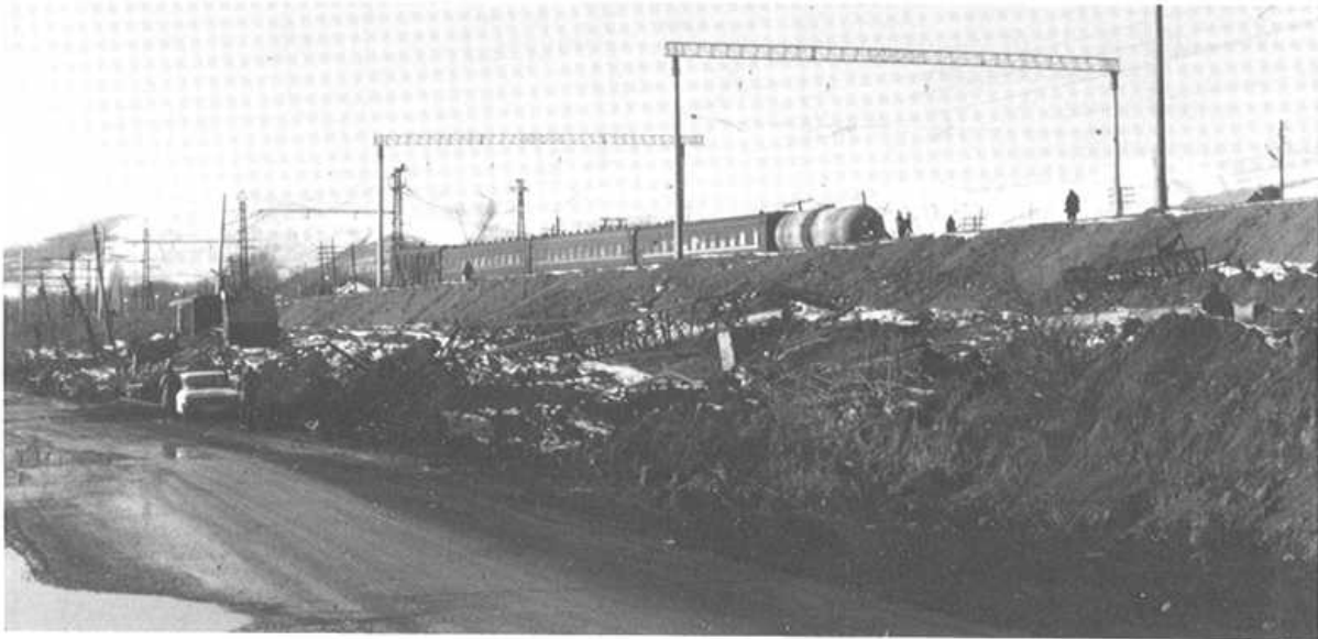
Main rail line at Nalband between Leninakan and Spitak. Ties, rails, and overhead components damaged by massive landslide had been replaced and service restored at time photograph was taken. Part of the landslide debris has been moved to roadside.
