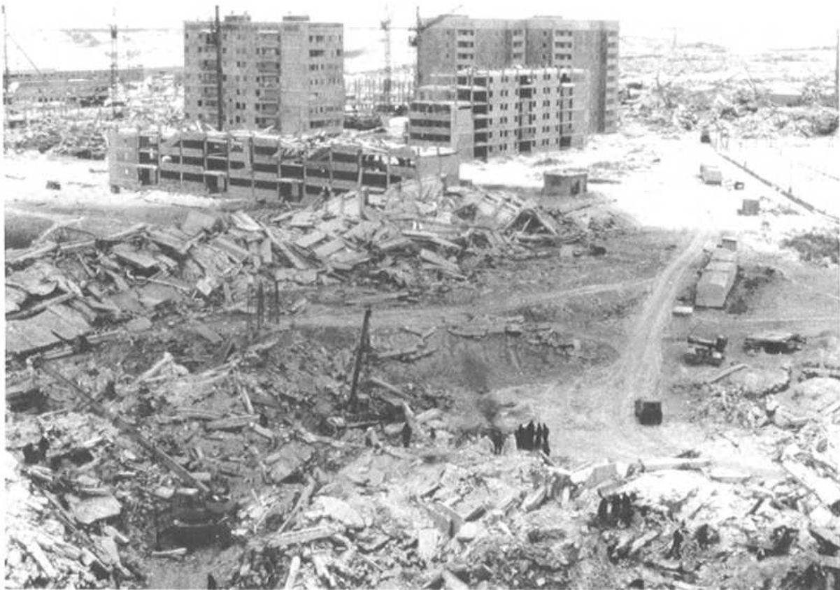
In Leninakan the tall large-panel structures under construction in background sustained little damage. Foreground has wreckage of several nine-story precast-concrete-frame structures. (Photo courtesy of T. O'Rourke.)
