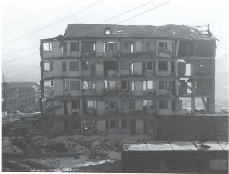
Remains of a five-story precast-concrete-frame residential building in Spitak.
