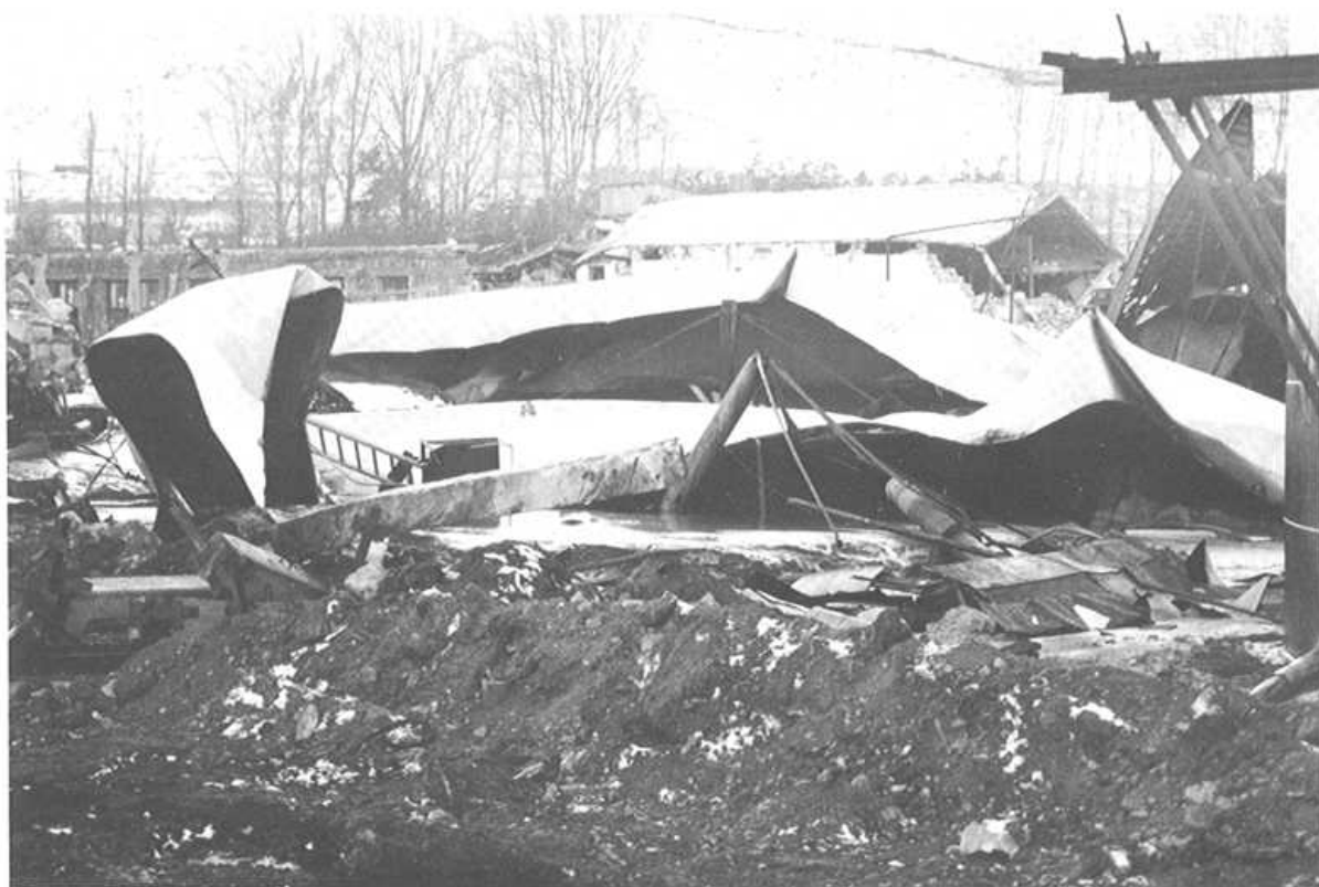
Spitak Sugar Refinery: Unanchored and corroded vertical tanks that had probably contained liquids collapsed or sustained severe damage and lost their contents.
