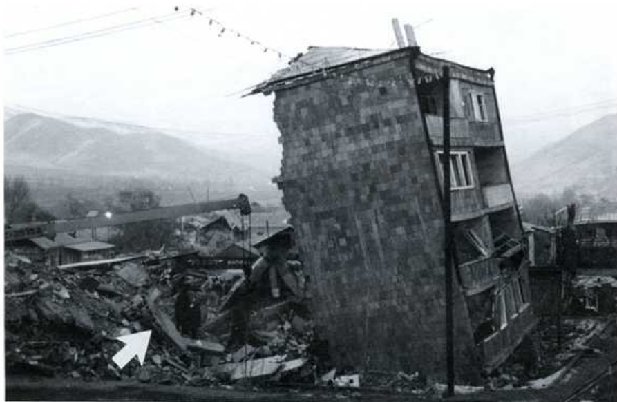
Remains of an unreinforced masonry structure with precast elements in Spitak. Arrow indicates hollow-core floor plank in rubble.
