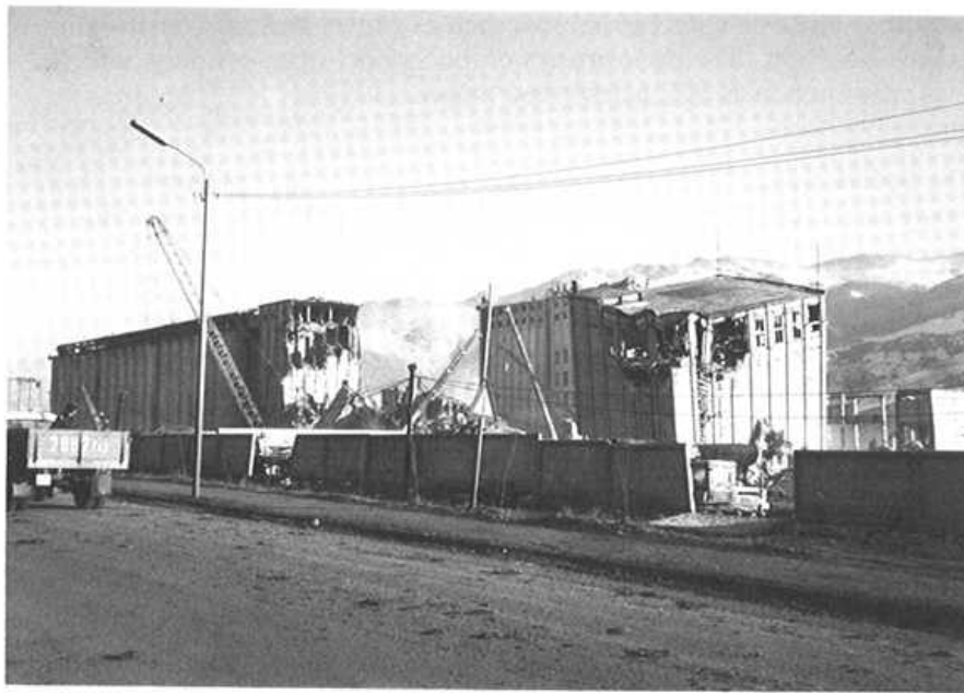
Standing remnant of precast-concrete furniture factory in Leninakan. It was reported that over 300 workers were killed in the collapsed sections of this structure.
