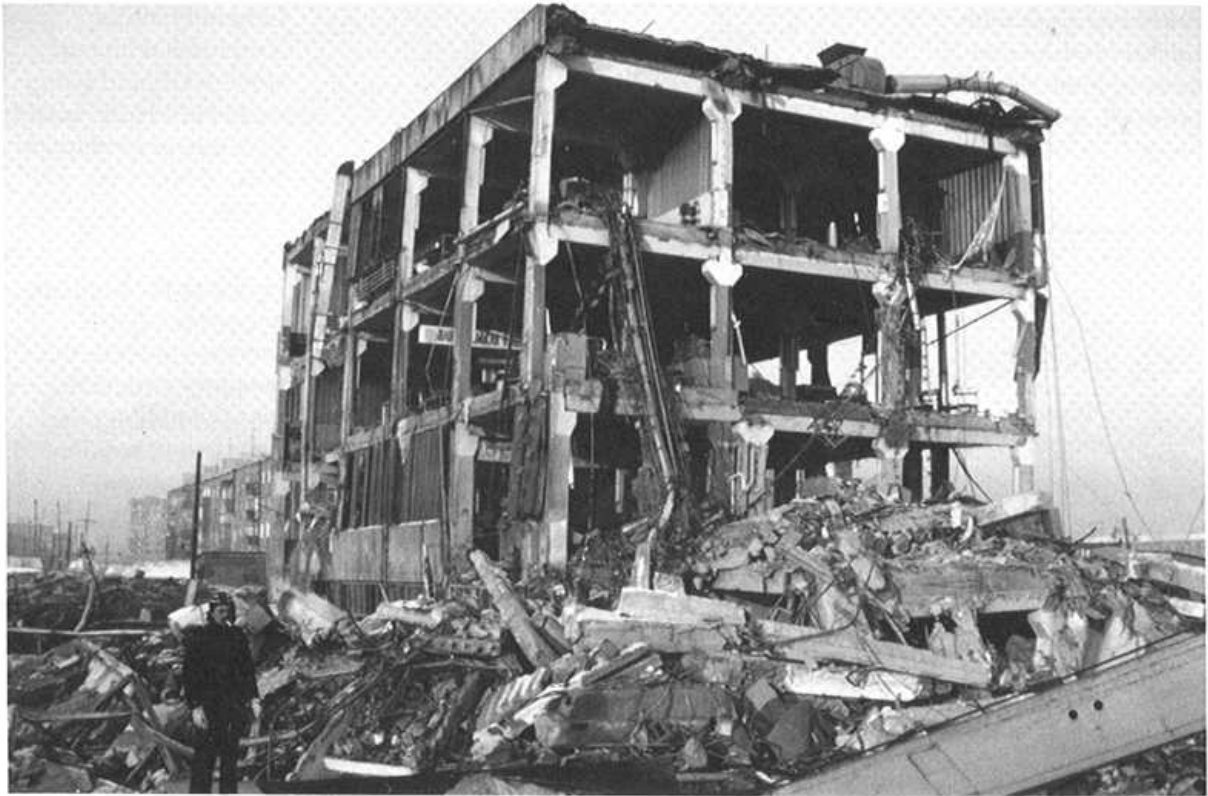
Standing remnant of precast-concrete furniture factory in Leninakan. It was reported that over 300 workers were killed in the collapsed sections of this structure.
