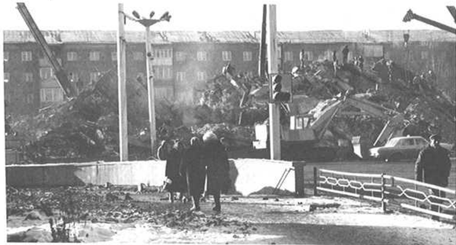
Collapsed 10-story lift-slab building. In foreground, entrance to a subterranean walkway that was undamaged.
