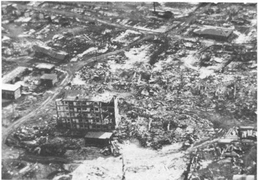
Contrasting earthquake effects on similar types of multi-story building clusters in Kirovakan at top and Spitak at bottom. (Photos courtesy of L. Cluff.)
