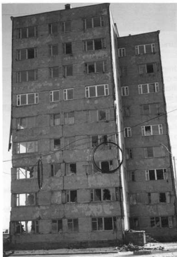
Rubble of several collapsed precast-concrete-frame buildings in Leninakan in the foreground. A structure of the same design in the background.
