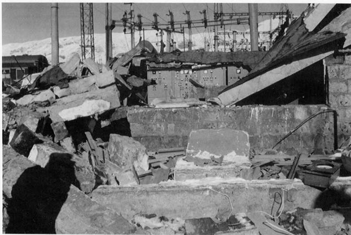
Nalband Electric Substation: Equipment that apparently remained intact or had limited damage within collapsed control building. Electrical control cabinets supporting roof fragment (top), medium-voltage metal-clad switchgear (bottom).
