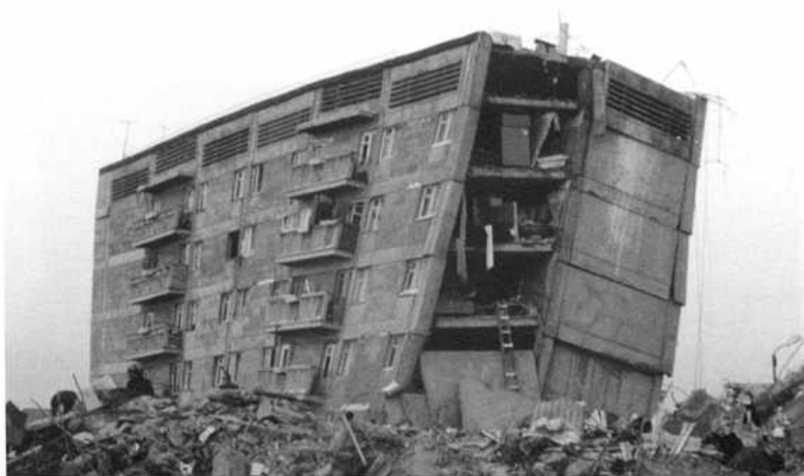
Rubble of several collapsed precast-concrete-frame buildings in Leninakan in the foreground. A structure of the same design in the background.
