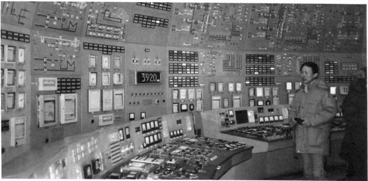
Armenia Nuclear Plant: Unit 2 control room. The panel indicates that unit was operating at 392 MW, approximately 90% of capacity, during U.S. investigation two weeks after earthquake.
