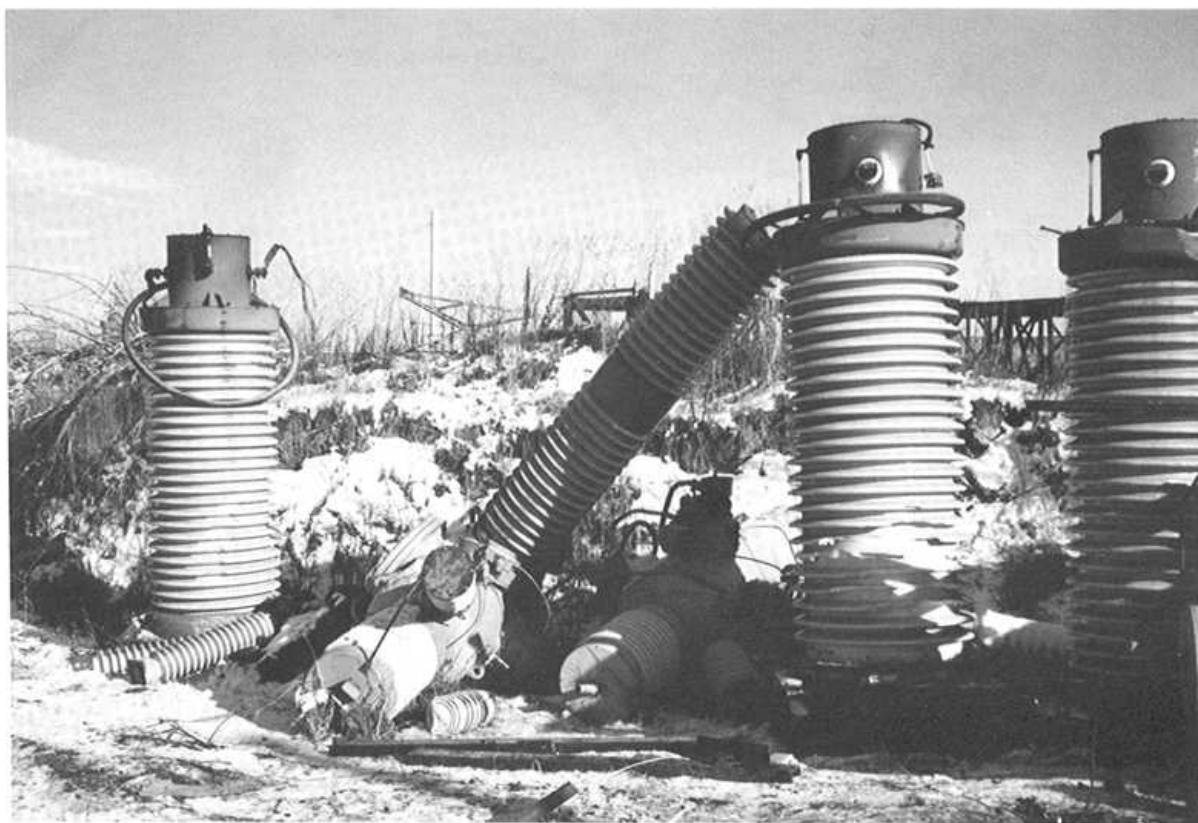
Leninakan-2 Electric Substation: Damaged ceramics in the 220 kV yard.
