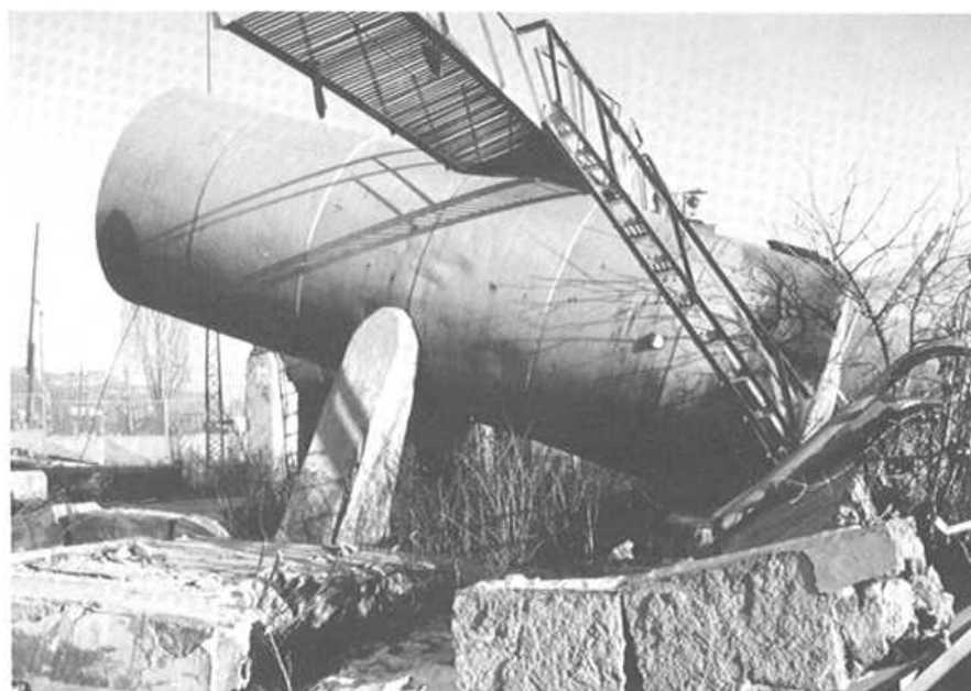
Spitak Sugar Refinery: Unanchored and corroded vertical tanks that had probably contained liquids collapsed or sustained severe damage and lost their contents.
